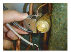
Remove the SOLENOID COIL.
