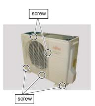
Remove the mounting screws.
