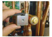
Remove the SOLENOID COIL.
