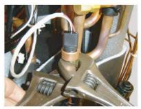
Remove the PRESSURE SENSOR with wrench. Note the tightening torque at the installation. Tightening torque is 12±1.5N•m.
