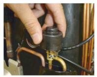
Remove the EEV coil by hand.
