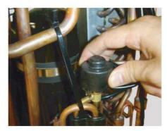
Remove the EEV coil by hand.
