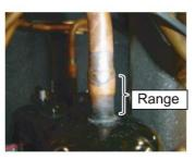
Cut the Suction pipe in this range. Remove the COMPRESSOR.
