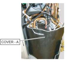
Remove the COVER-A,-B and -C.
